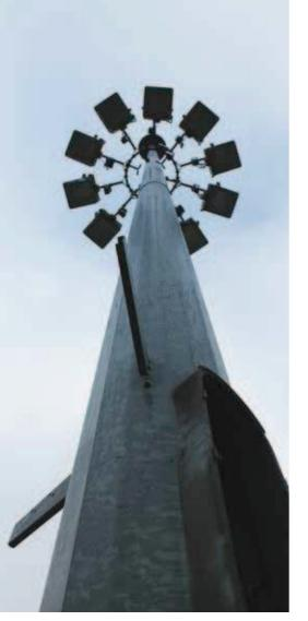
Designed by PETITJEAN, CM 61, 10 and 20 mobile rings are manufactured to support a large number of floodlights, allowing maintenance on the ground level while guaranteeing a high level of security.
